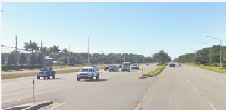
Existing: US 41 and Ridge Drive
