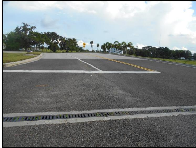
**Figure 3: 23<sup>rd</sup> Street West, Crest Vertical Curve at Intersection Approach**
