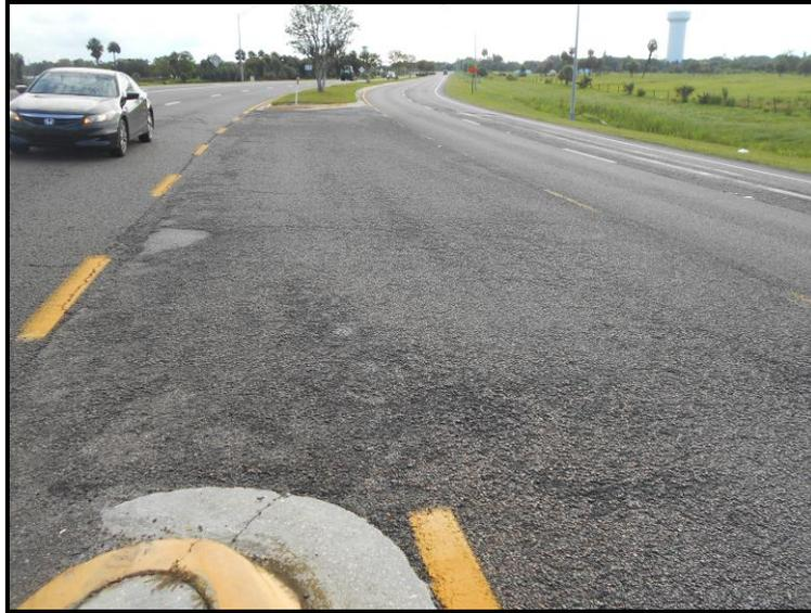
**Figure 5: Existing Intersection Pavement Condition**
