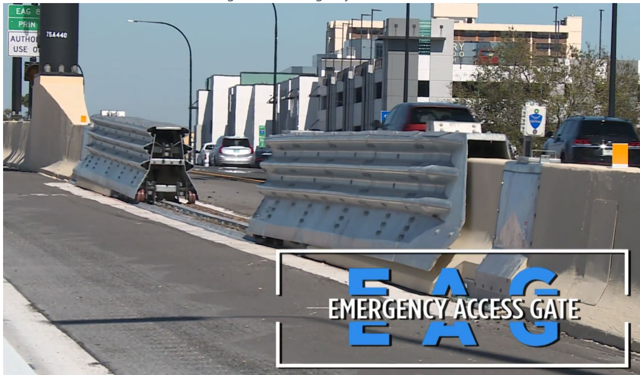
Figure 2-3: Emergency Access Gate
