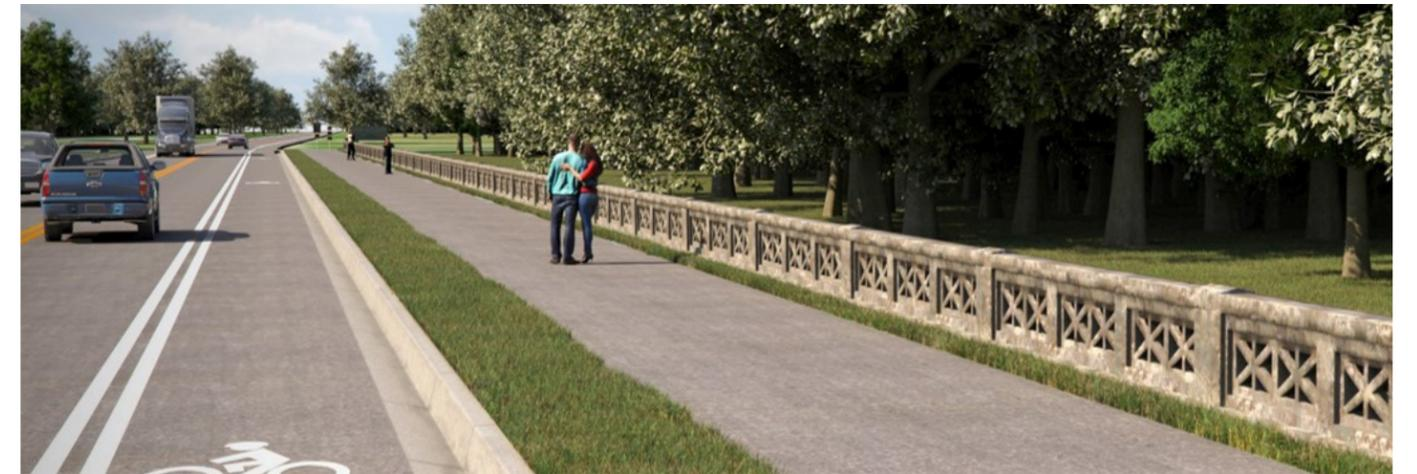
The existing bridge railing is planned to be repurposed. The project will evaluate bridge railing alternatives for the new bridge to mimic the pattern of the current railings while maintaining safety standards.
