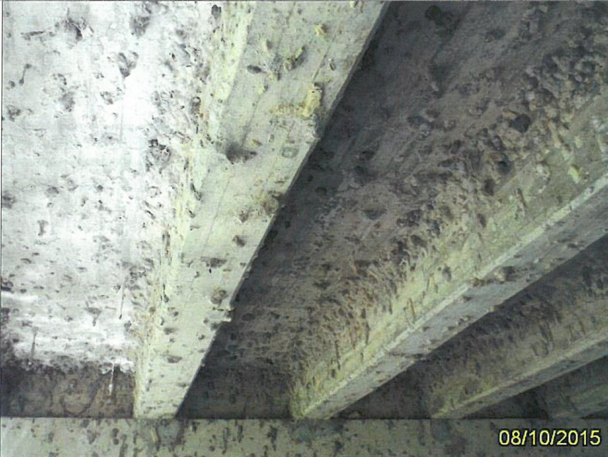
**Photo 1 - Elements 13 Unp Conc Deck/AC Ovl & 110 R/Conc Open Girder**
