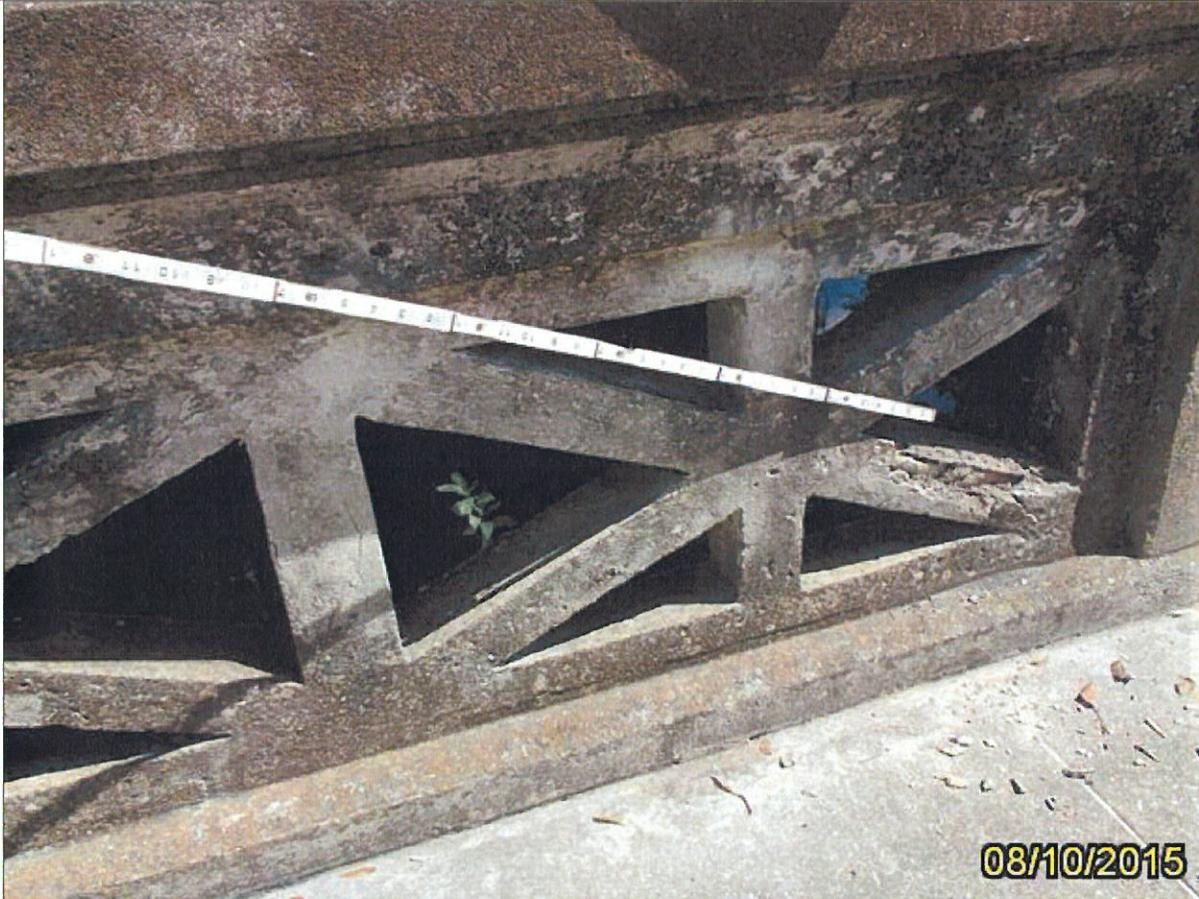
**Photo 4 - Element 331 Conc Bridge Railing**
