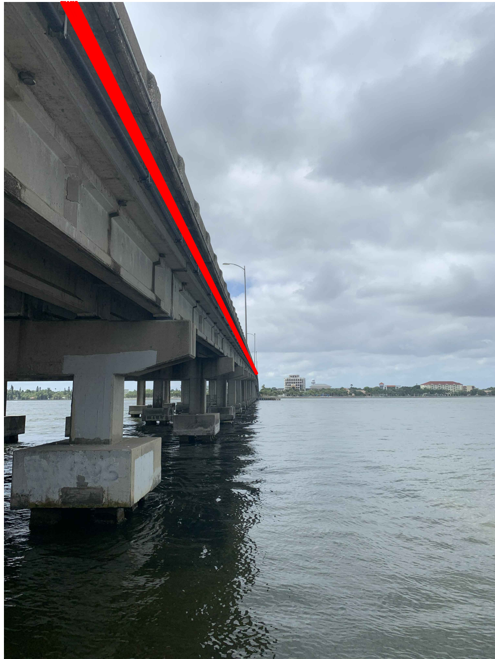
WEST SIDE – LOOKING SOUTH
