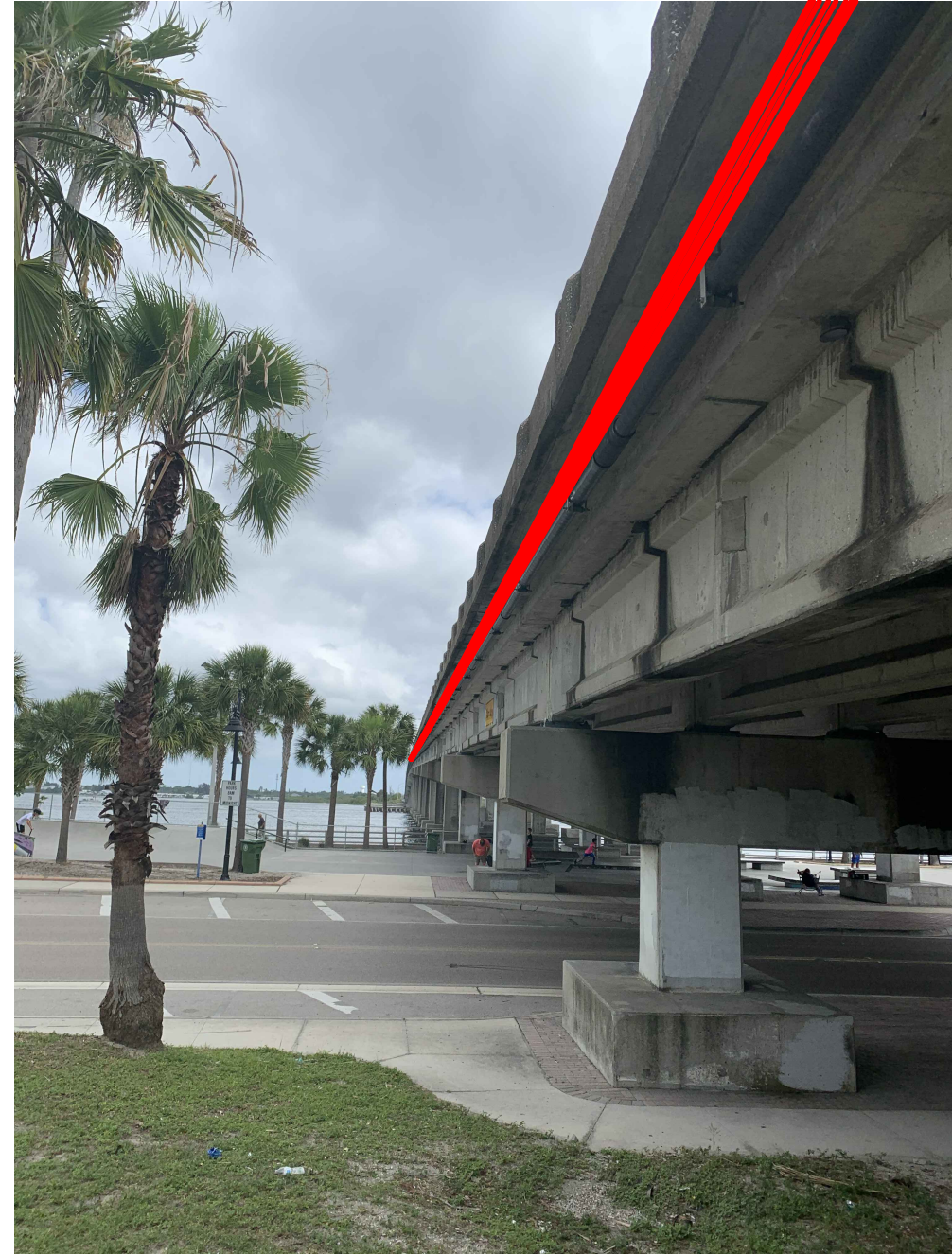
WEST SIDE – LOOKING NORTH
