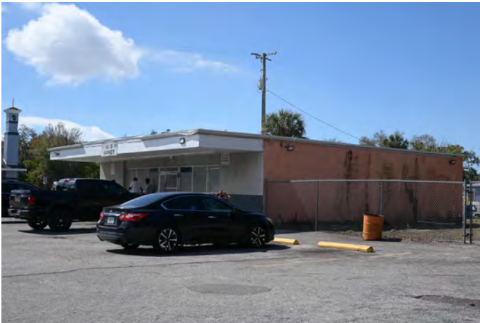
8MA03123_c Facing SW
