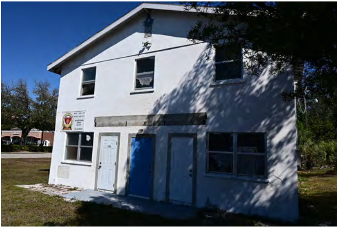
8MA03135_c Facing NE
