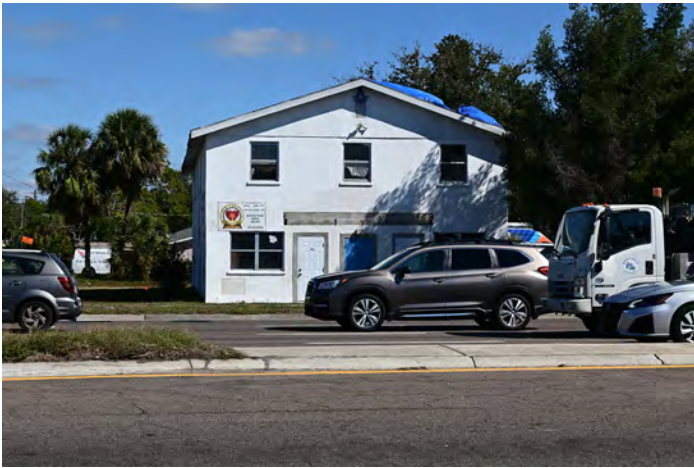
8MA03135_a Facing E
