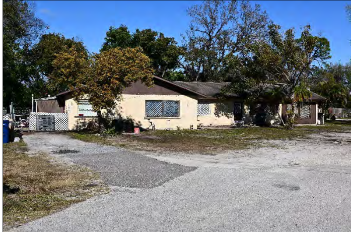
Figure 42. Resource 8MA03141, view facing northeast.
