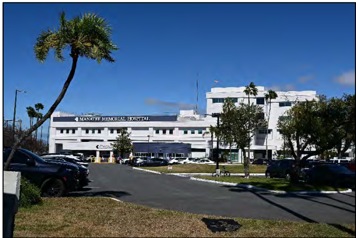
Figure 22. Resource 8MA02569, view facing north.
