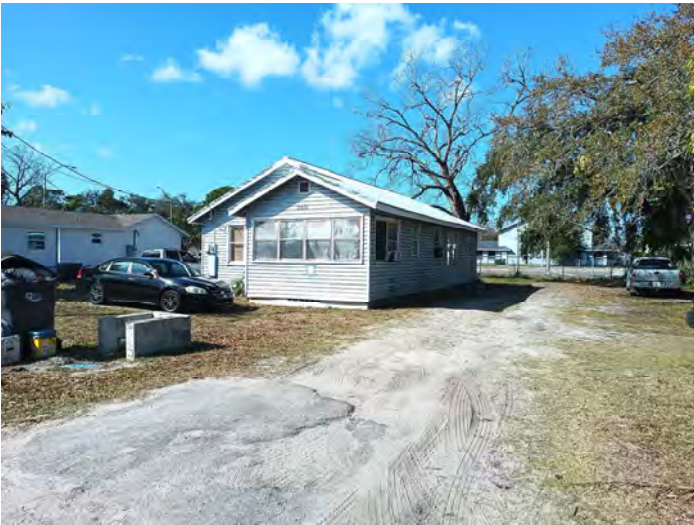
8MA03125_c Facing SW
