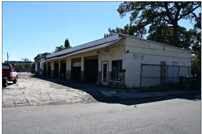
Figure 35. Resource 8MA03134, view facing southwest.
