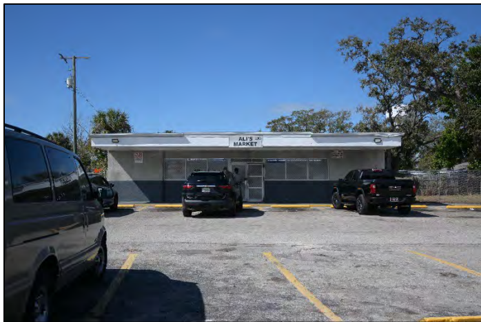
Figure 24. Resource 8MA03123, view facing west.
