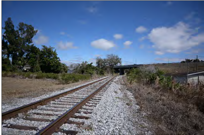
Figure 44. Resource 8MA01381, view facing northeast.
