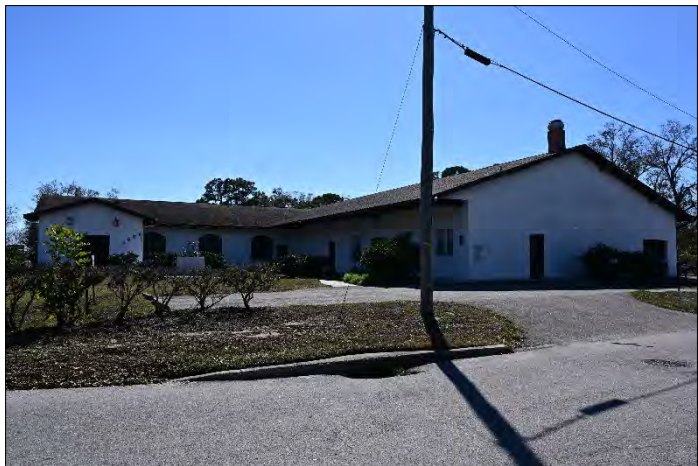
Figure 34. Resource 8MA03133, view facing southwest.
