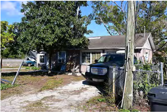
8MA03140_c Facing NE
