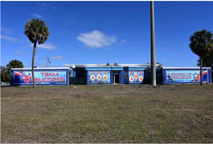
8MA03136_a facing E
