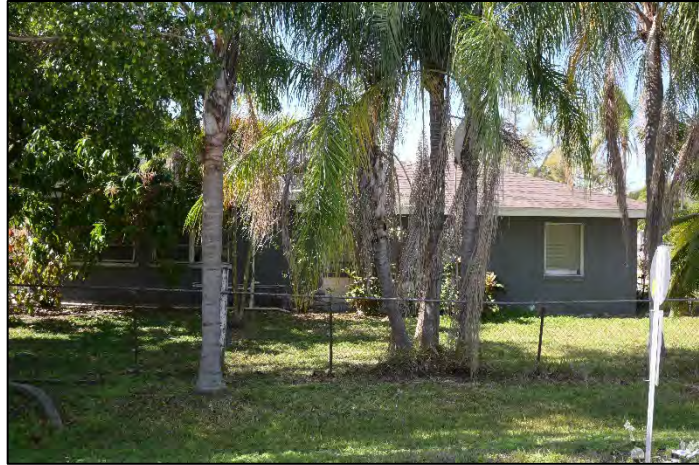
Figure 28. Resource 8MA03127, view facing west.
