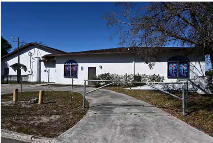
8MA03133_e Facing N
