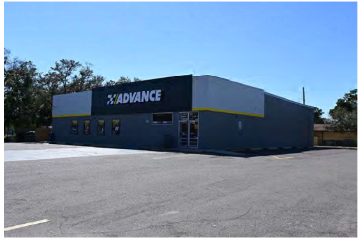
8MA03131_d Facing SW
