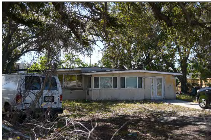
Figure 23. Resource 8MA03122, view facing southwest.
