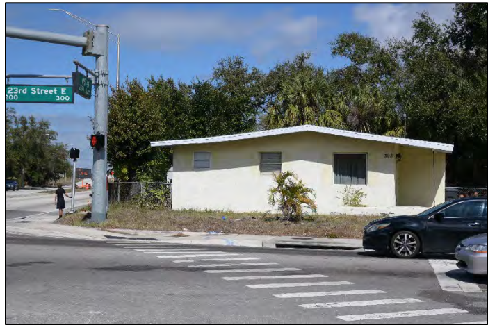
Figure 25. Resource 8MA03124, view facing north.
