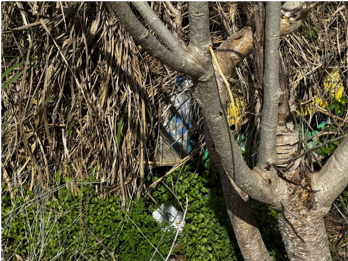
CD-9 24" RCP at US 41 Station 269+09 facing west
