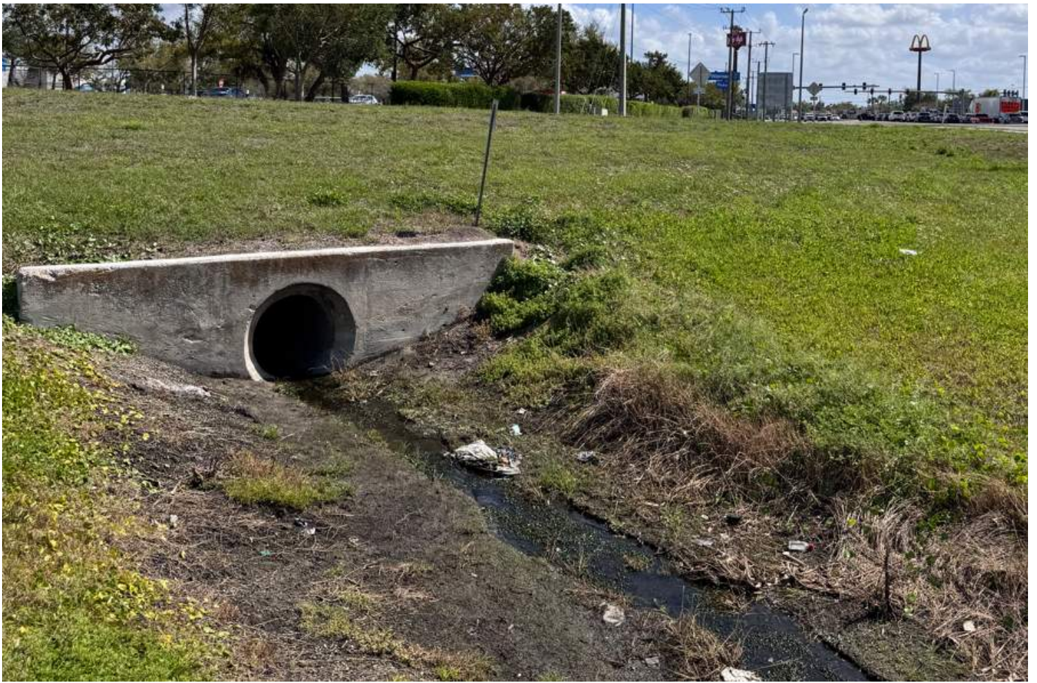
CD-8 30" RCP at US 41 station 259+86 facing northeast
