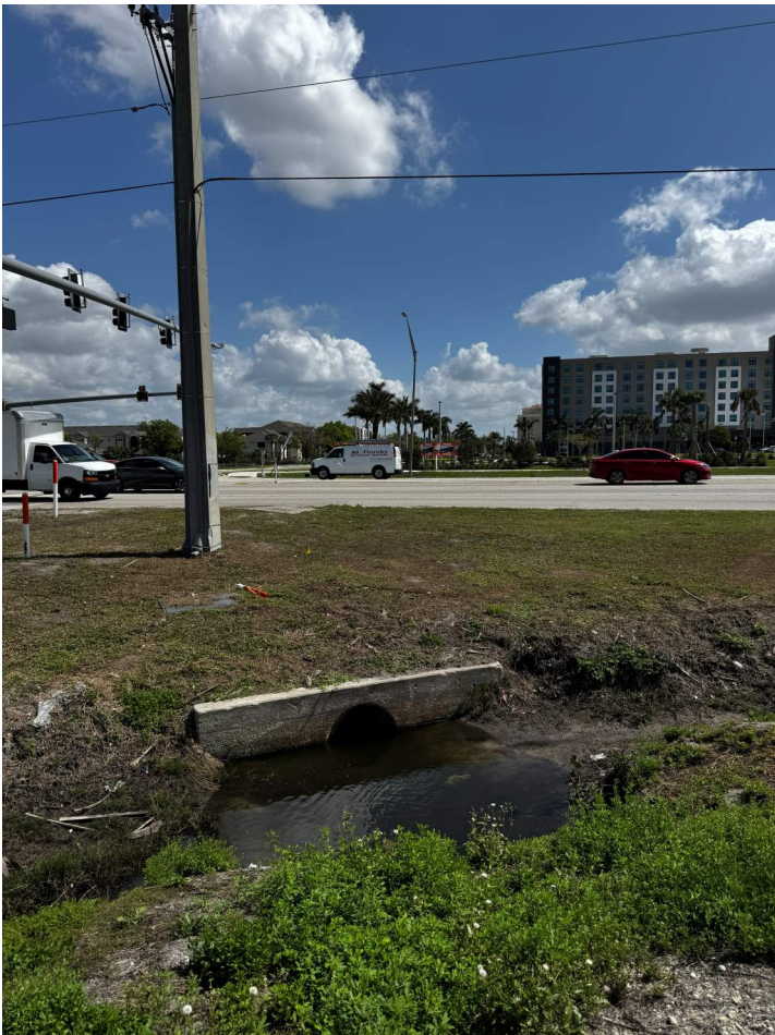
CD-2 24" RCP at US 41 station 242+37 facing east
