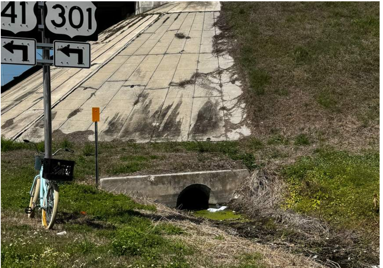
CD-6 30" RCP at US 41 station 258+21 facing west
