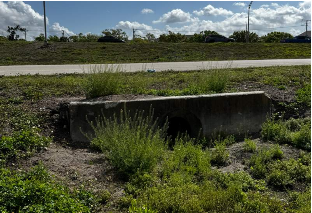
CD-4 24" RCP at US 41 station 252+07 facing east
