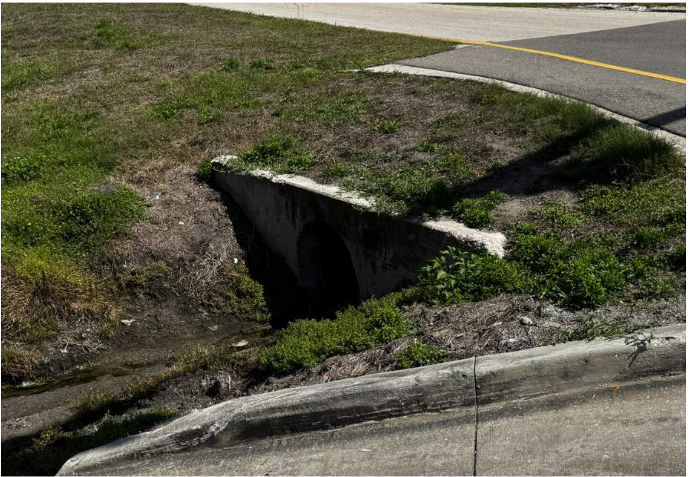
CD-7 30" RCP at US 41 station 258+87 facing northeast
