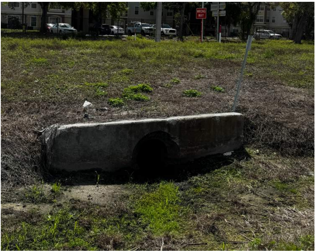
CD-3 24" RCP at US 41 station 251+00 facing east
