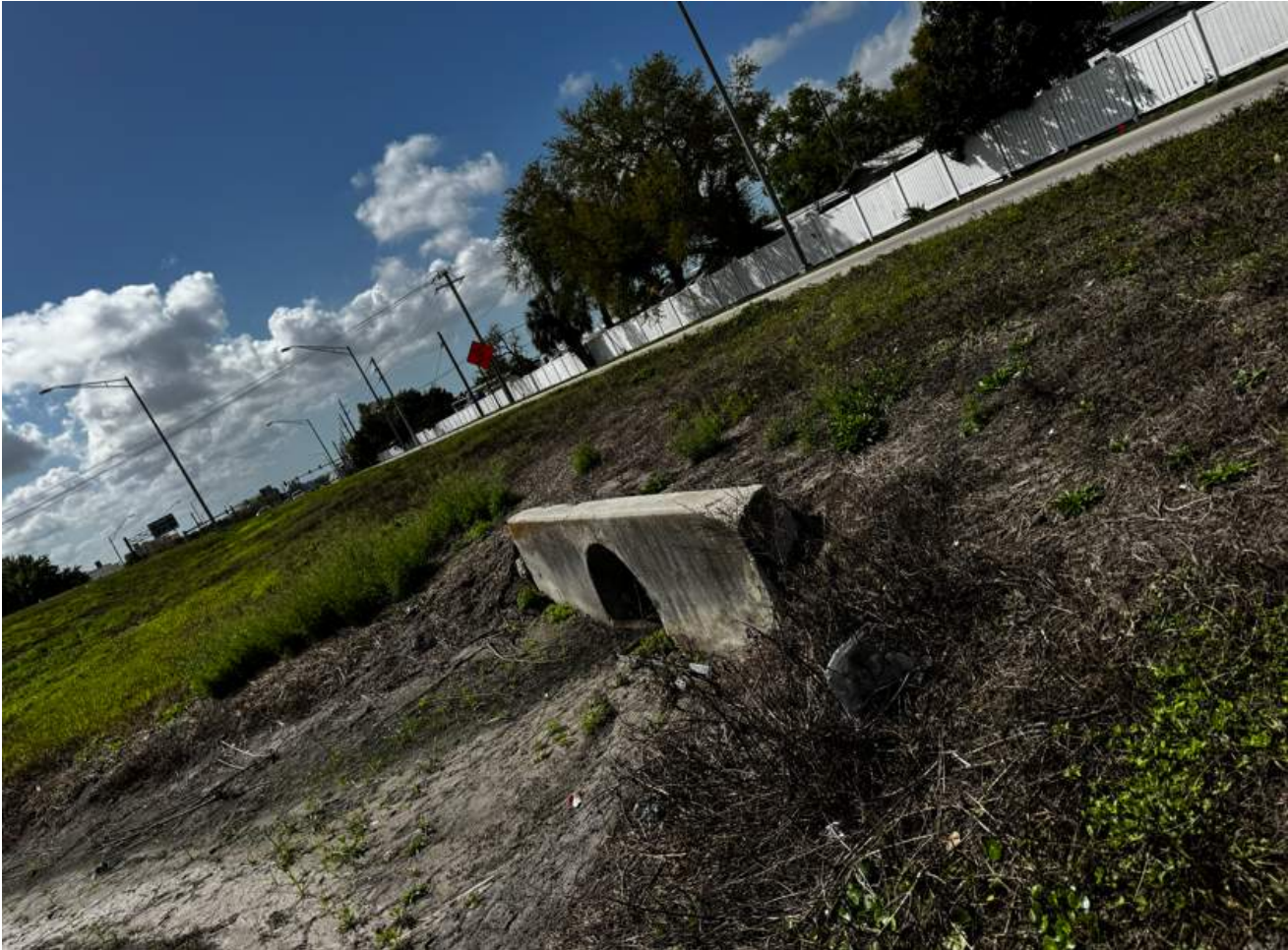
CD-4 24" RCP at US 41 station 252+07 facing southwest
