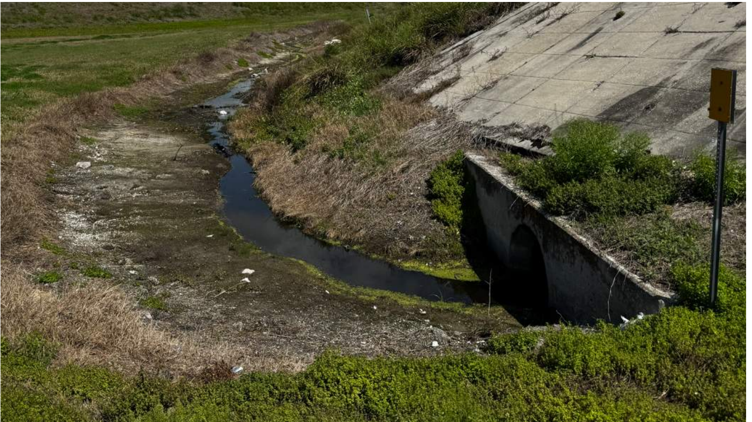
CD-6 30" RCP at US 41 station 258+21 facing north
