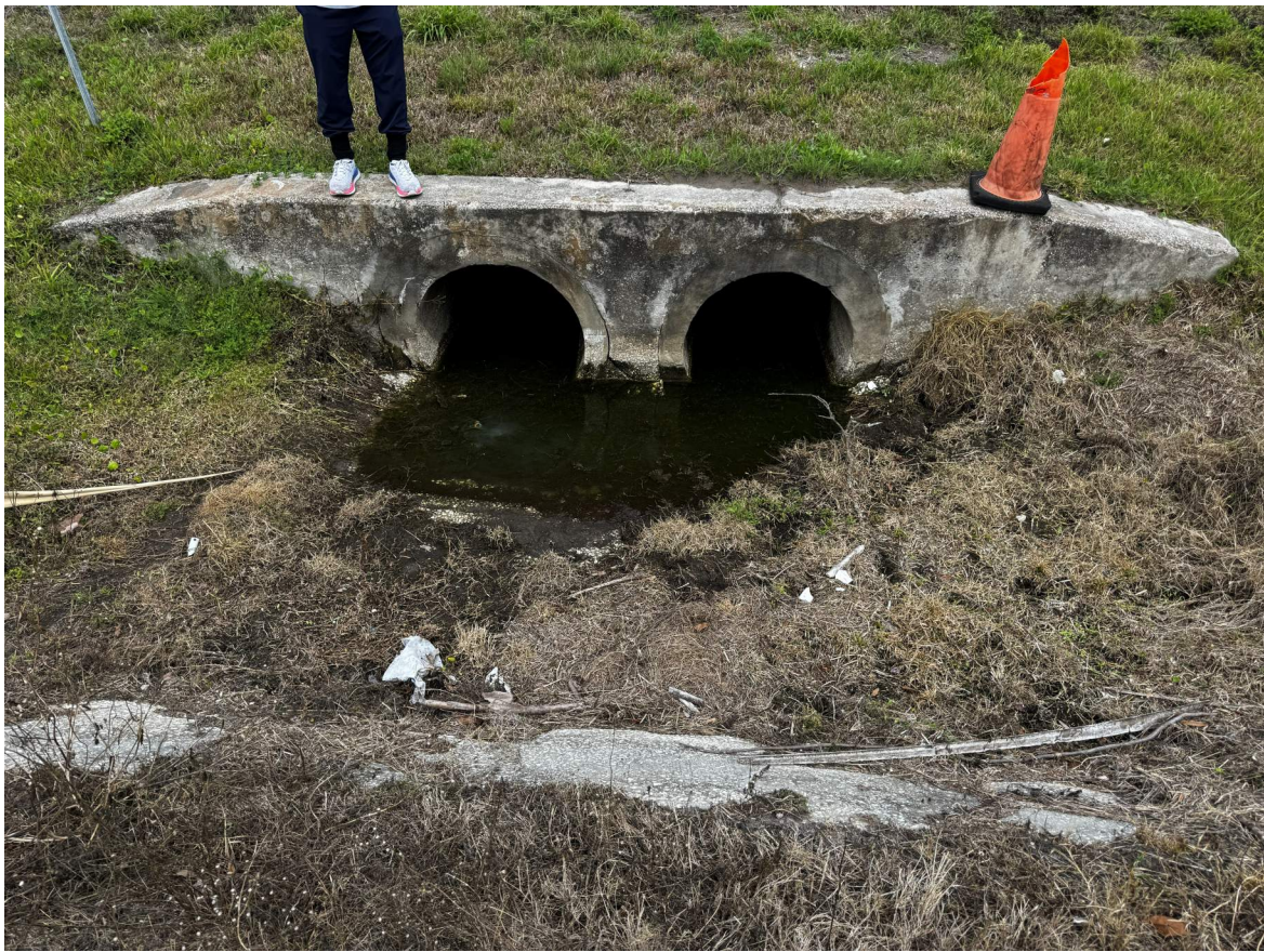
CD-1 2-36" RCP at US 301 station 508+04 facing north
