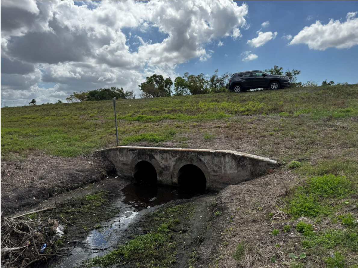
CD-1 2-36" RCP at US 301 station 508+04 facing south
