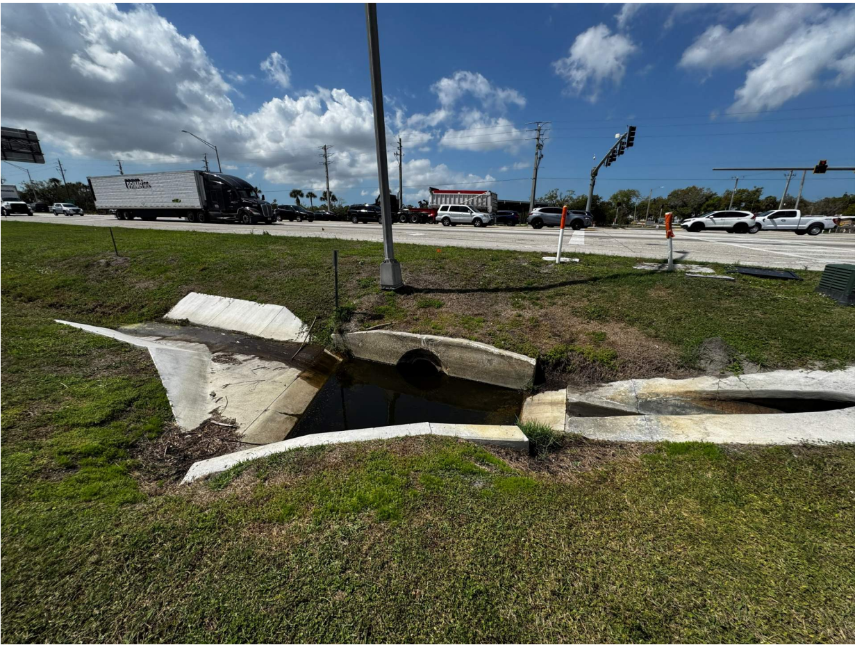
CD-2 24" RCP at US 41 station 242+37 facing west
