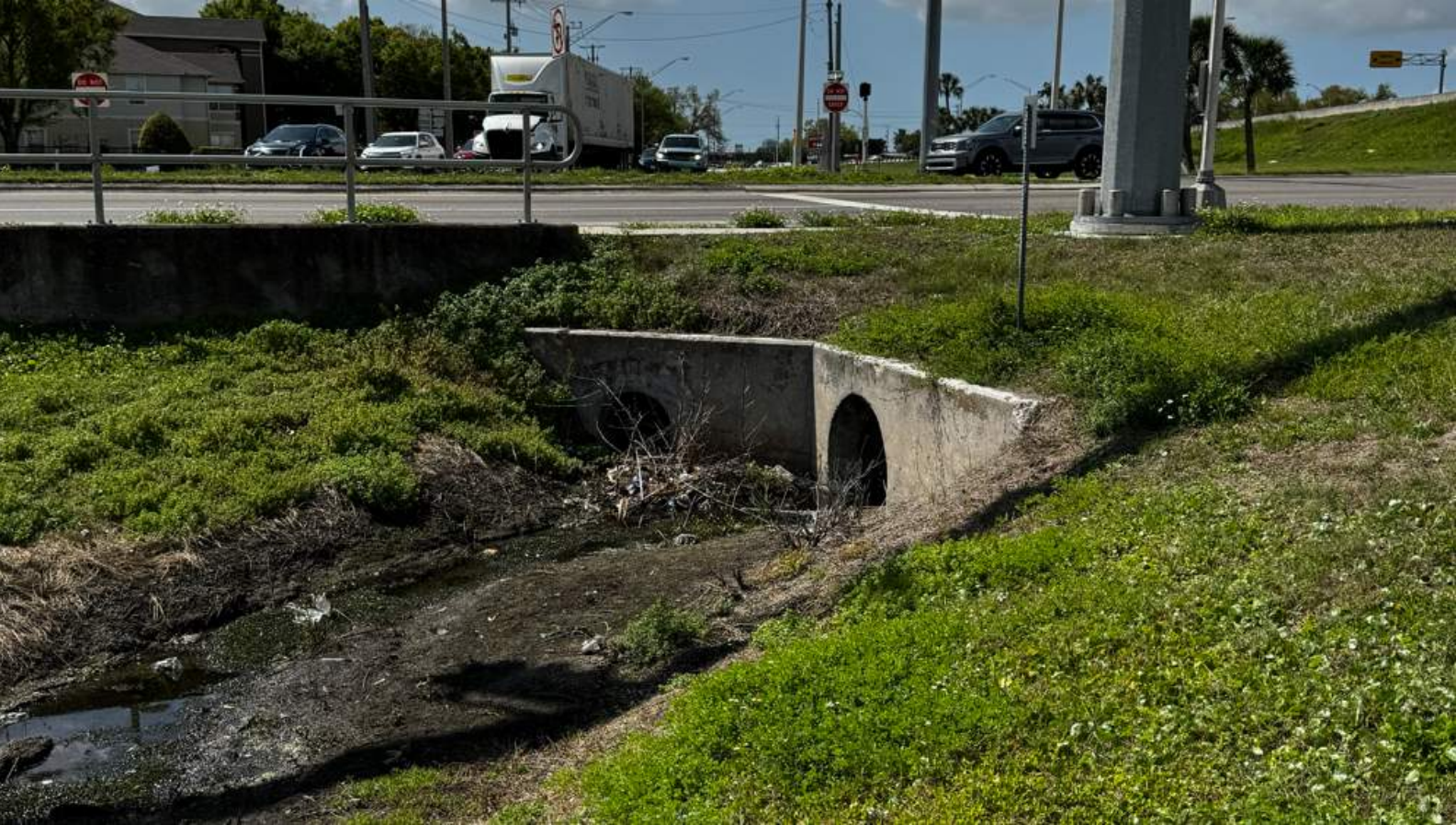
CD-7 30" RCP at US 41 station 258+87 facing south
