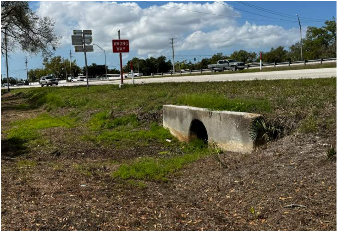
CD-3 24" RCP at US 41 station 251+00 facing southwest
