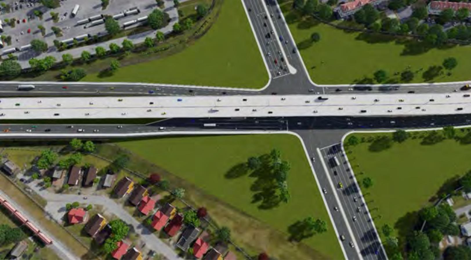
Figure 63: US 19/US 41 interchange elevated throughway option from above
