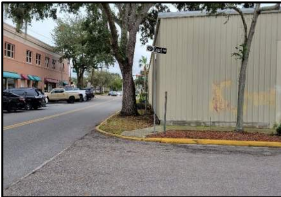
Photo 5 - Facing ROW south along Sixth Street, with large oak and utilities building.
