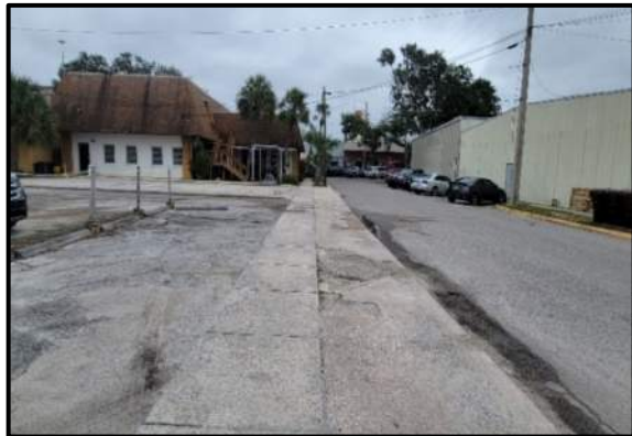
Photo 6 - Looking east at conditions along Court Avenue. Note the paved over ROW.
