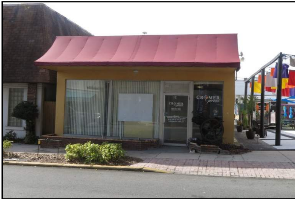
Photo 34 - 24 N 6th Street (8PO09908), looking west.
