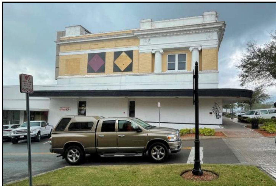
Photo 27 - Growers' Commercial Bank of Haines City (8PO09909), looking west.
