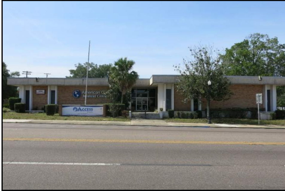
Photo 38 - 502 E Hinson Ave (8PO08323), looking south.
