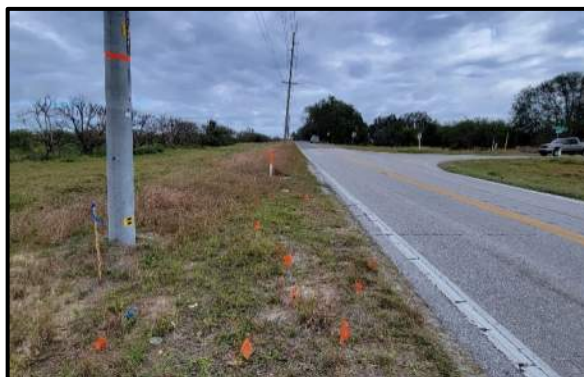
Photo 2 - View east of buried utilities/fiber cable in APE boundaries.
