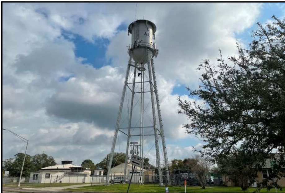
Photo 22 - Lake Alfred Water Tower (8PO04728), looking northeast.
