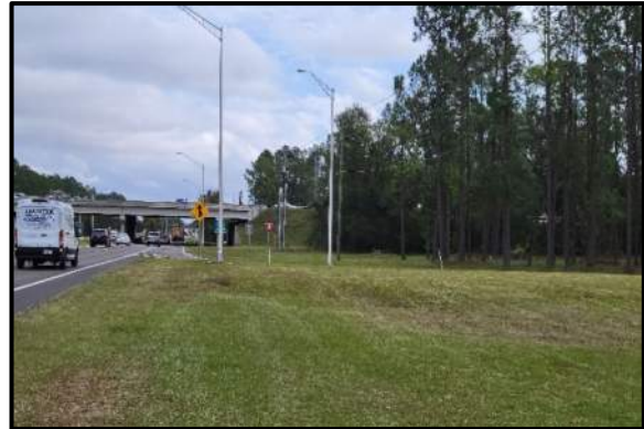
Photo 4 - Looking east at U.S. 27 overpass.
