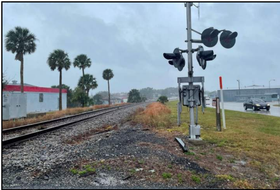
Photo 24 - South Florida Railroad (CSX RR) (8PO07219), looking south from E Main Street.
