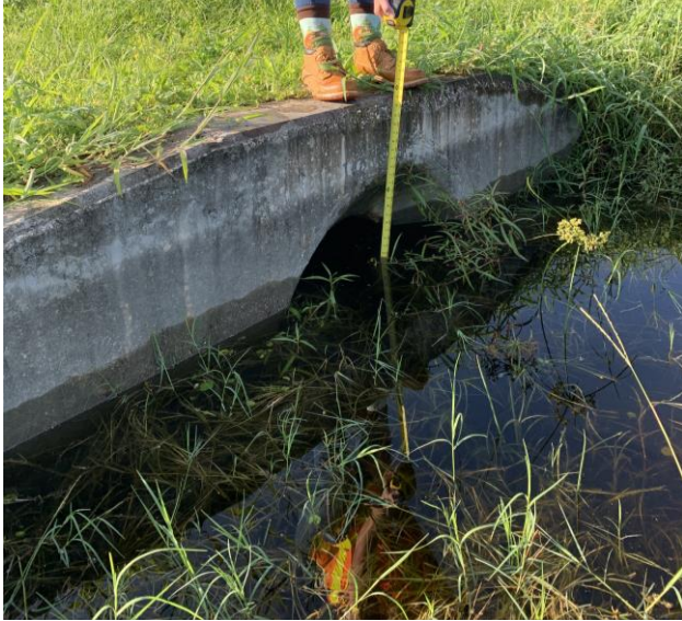
CD 12-01 Berkley Road and Deen Blvd. Single 18" RCP
