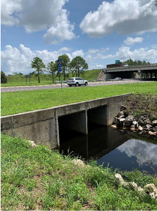
CD 12-19 US 17-92 approx. 250-ft west of US 27 Double 4' x 4' Box Culvert
