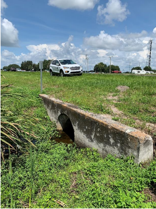
CD 12-15 US 17-92 approx. 1400-ft east of Sweetwater Club Blvd. Single 30" RCP
