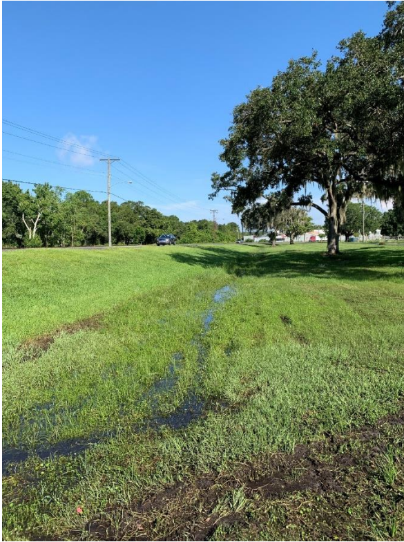
Ponding in ditch alongside Ramsgate Road adjacent to cross drain CD 12-07.
