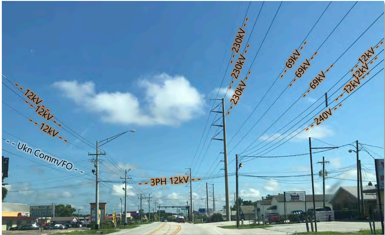
Figure 23: Photo of overhead utilities on Combee Road (looking north)
