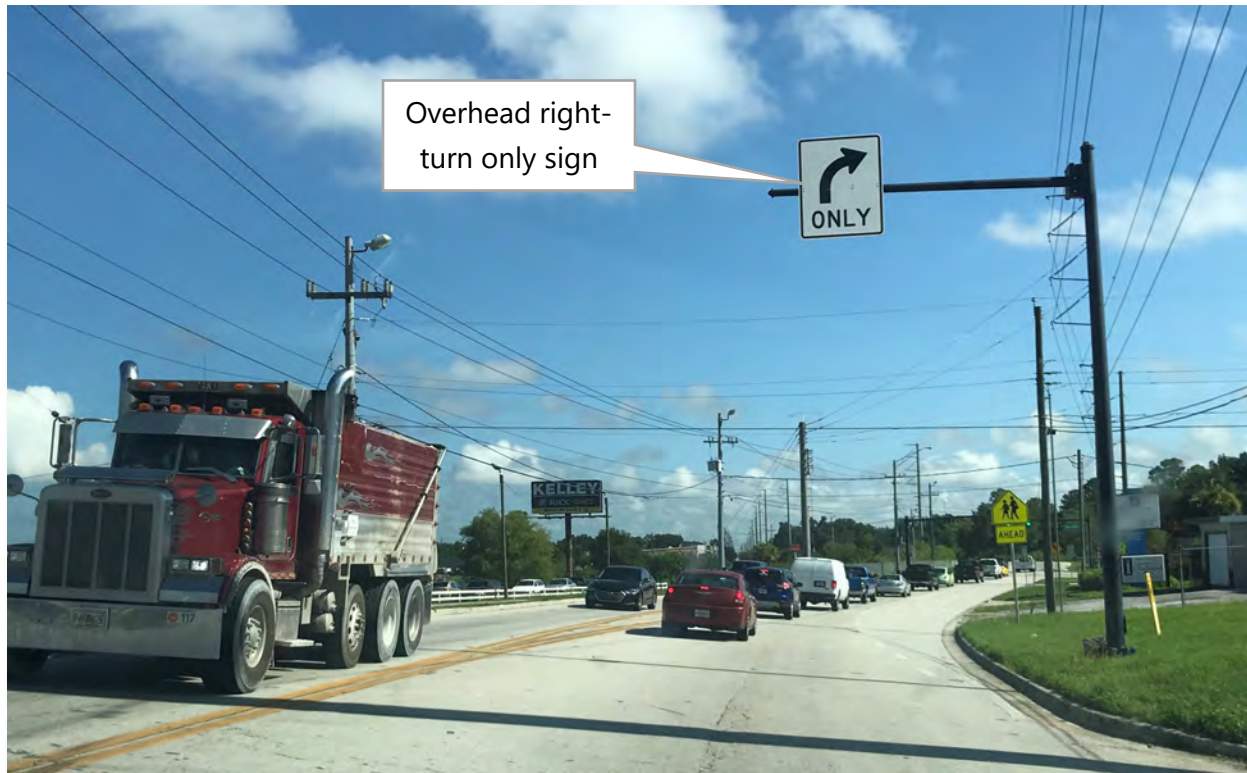
Figure 26: Photo of overhead sign structure on Combee Road (looking north)
