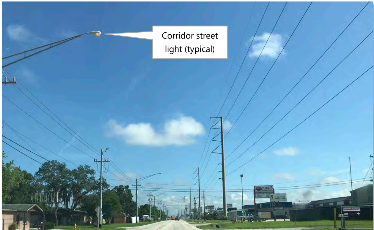
Figure 25: Photo of existing lighting along Combee Road (looking north)
