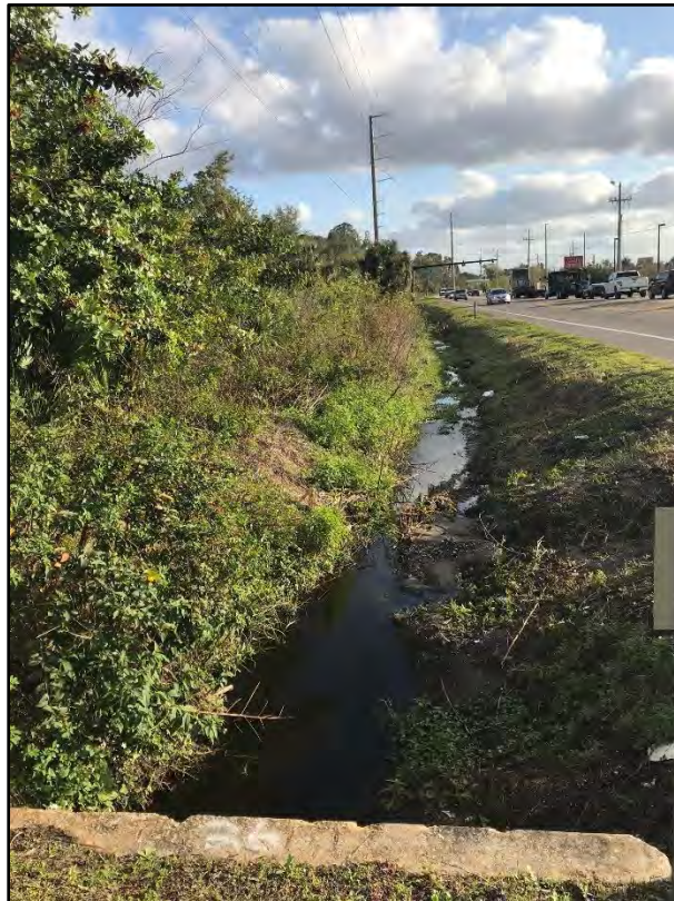
SW 01: West of SR 659 (Combee Road) facing south
