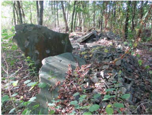
SMF-3: Concrete debris near west boundary
