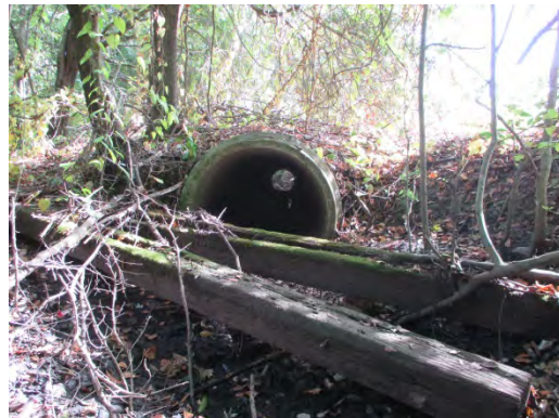
Railroad ties and drain pipe, south area
