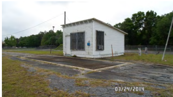
SMF-1: Northwest of scale house looking southeast
