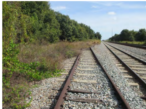
CSX railroad tracks along south boundary looking east
