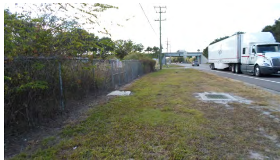
SMF-2: North boundary looking west
