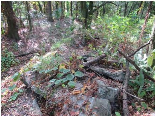
SMF-5: Concrete debris, west-central area
