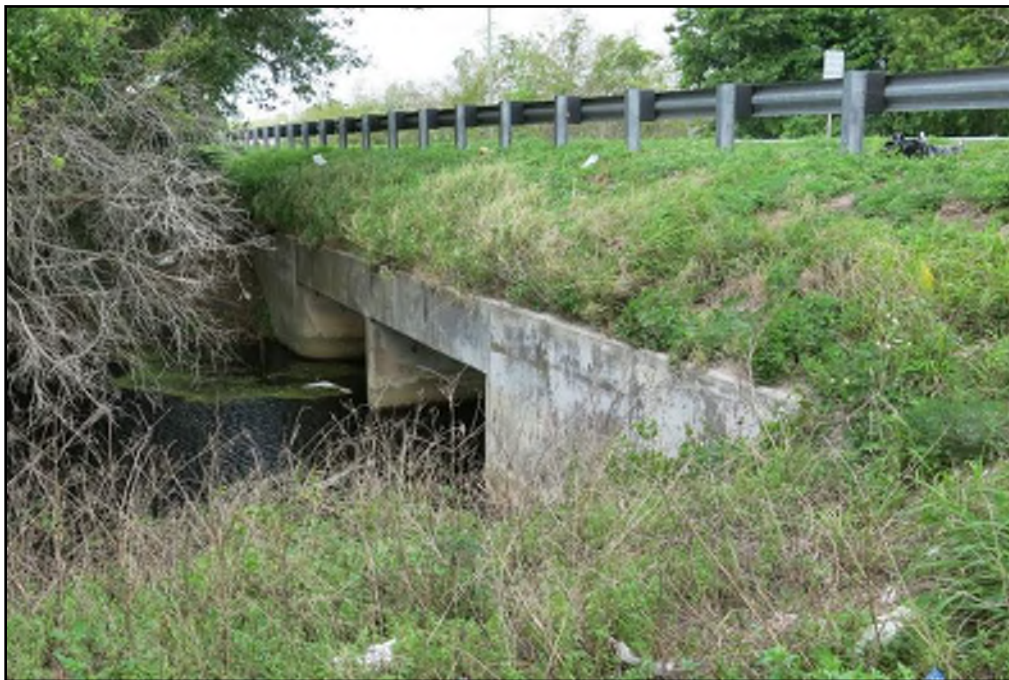
Photo 5.21. SR 544 over Lake Hamilton Creek (FDOT 160147) (8PO10087), looking northwest.
