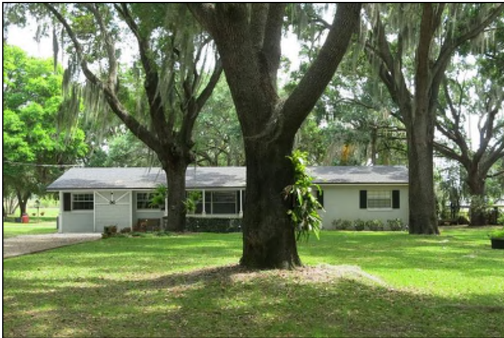
Photo 5.18. Ranch style building (8PO10053) located at 96 Hilltop Drive, looking east.
