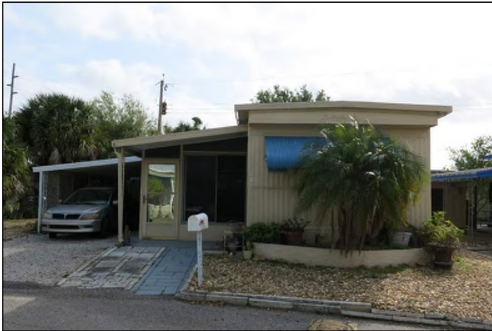
Photo 5.15. Mobile home with no style (8PO10060) located at 119 Ixora Drive, looking northeast.
