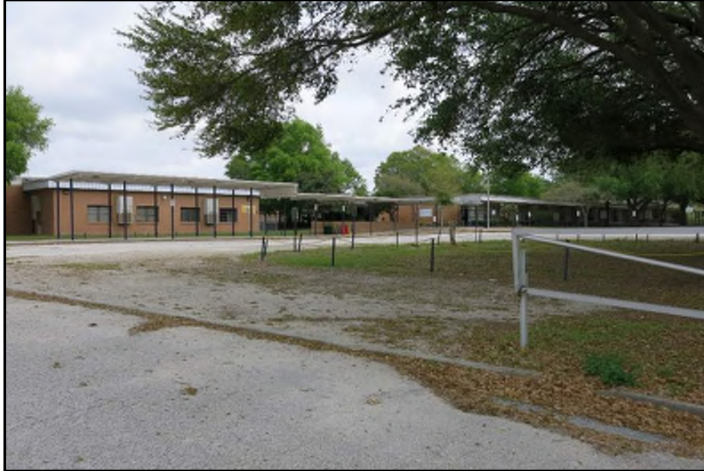
Photo 5.10. 801 Scenic Highway S/Alta Vista Elementary School (8PO10093; 8PO10094 and 8PO10095), looking northeast.
