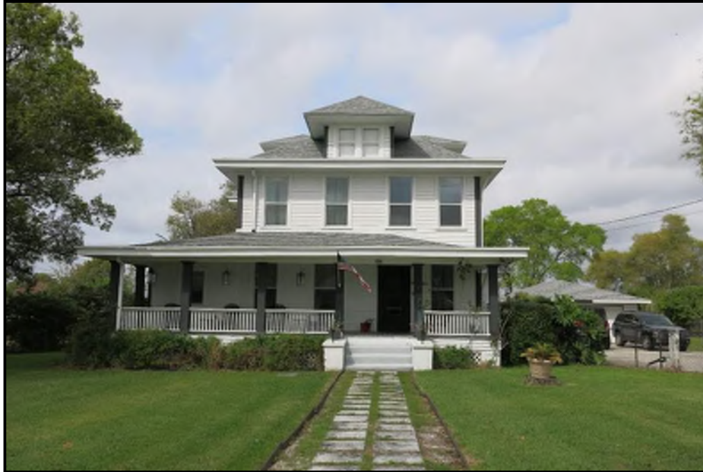
Photo 5.8. 2208 Peninsular Drive (8PO03077), looking west.
