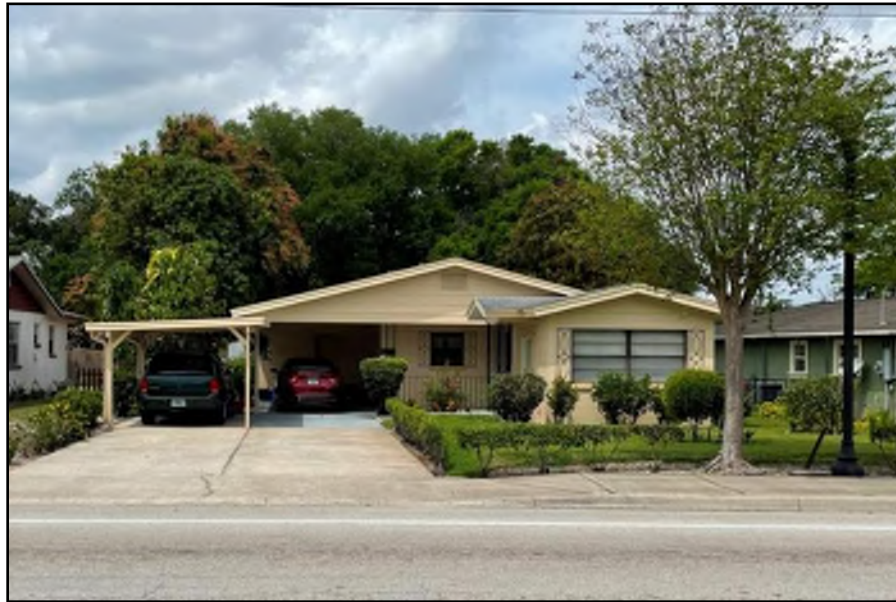
Photo 5.11. Masonry Vernacular style building (8PO10024) located at 2209 Lucerne Park Road, looking northwest.
