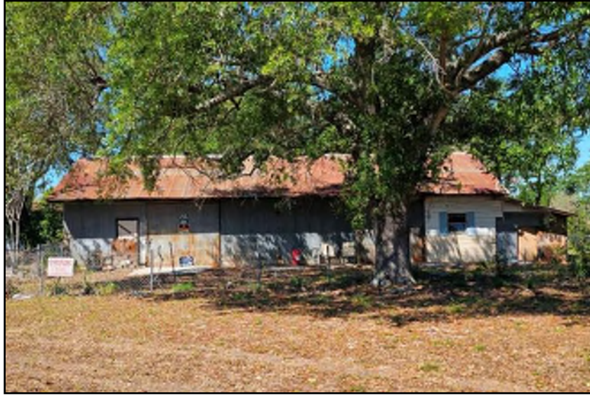
Photo 5.19. Industrial Vernacular style building (8PO10005) located at 2101 1st Street N, looking west.
