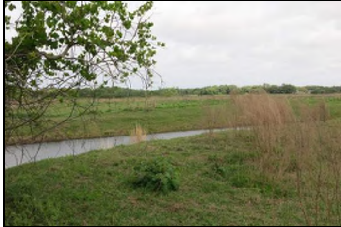
Photo 5.4. View of 8PO05047 (Lake Tracy Canal) facing northwest.
