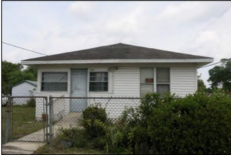
Photo 5.13. Frame Vernacular style building (8PO10016) located at 101 Avenue V NW, looking north.
