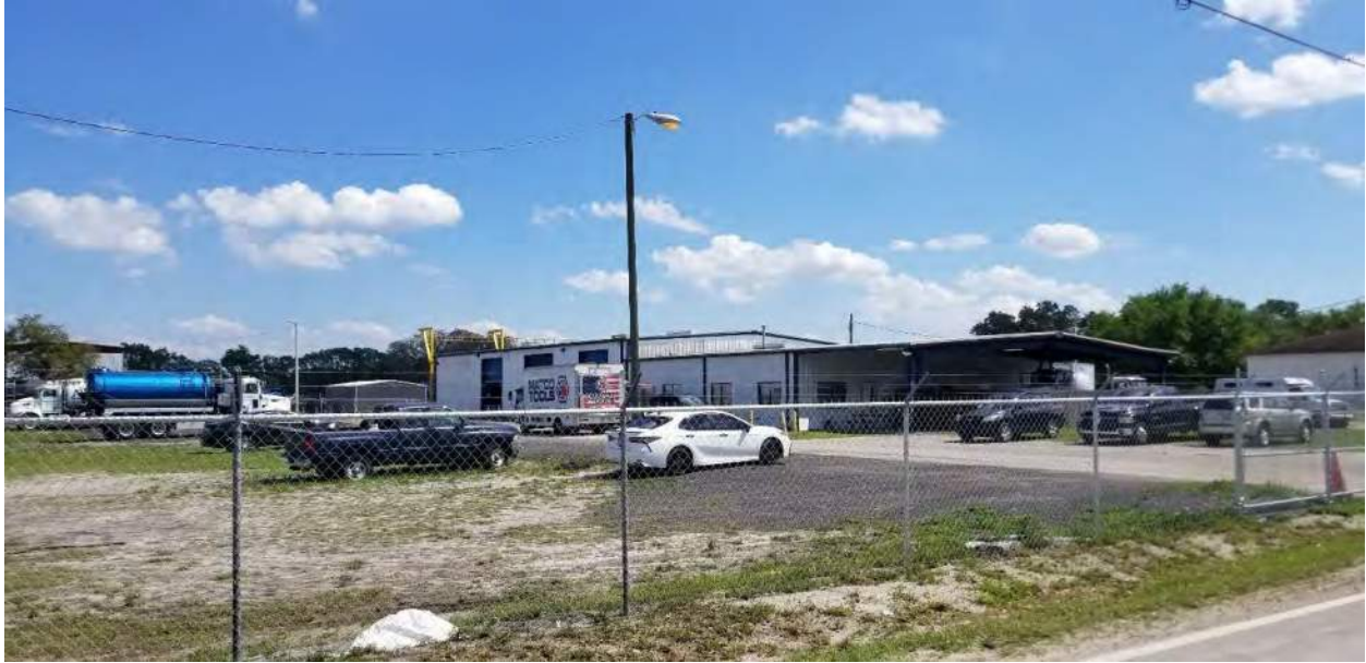
Photograph 25 Site 45 Synergy Recycling
