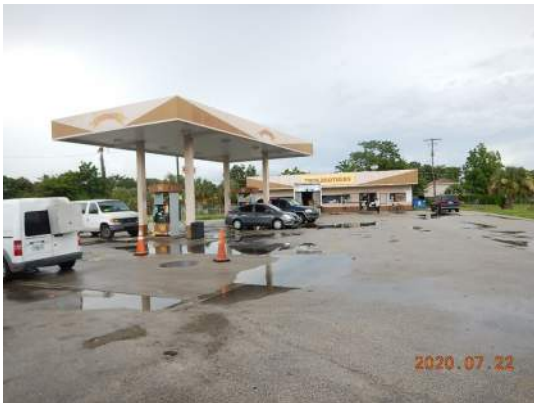
2020-07-22 General Site Photo
